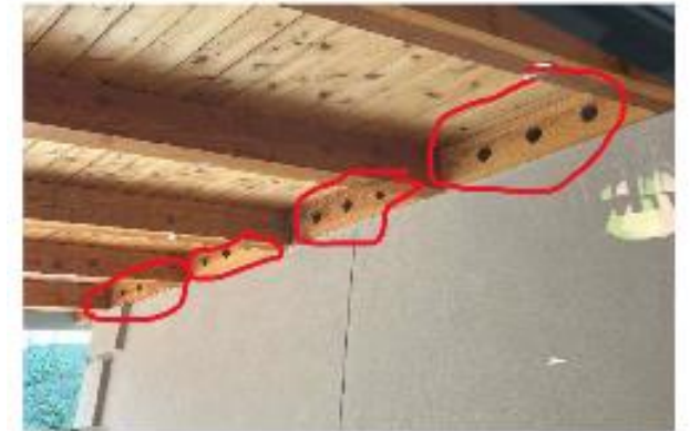
(Eave vents in combustible roof support structure, Admin. Building)
